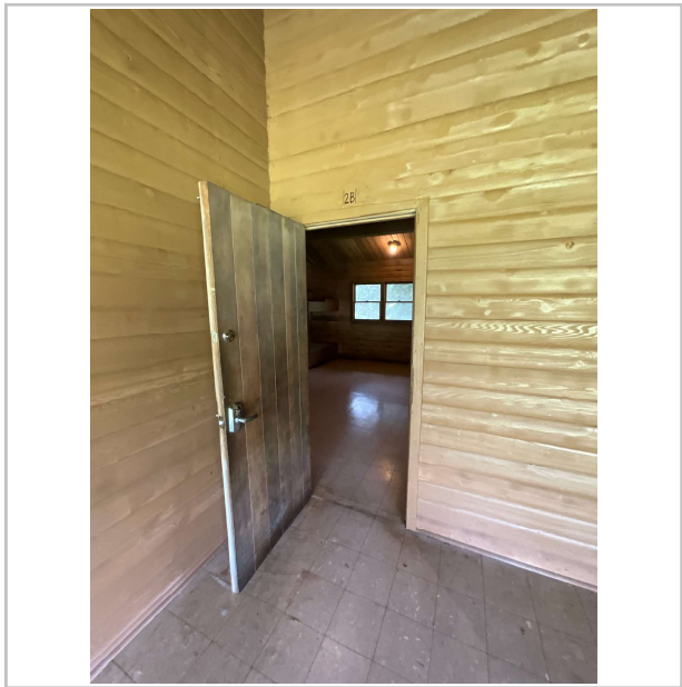
Cabin 2B Remove and replace interior VCT in bathrooms and main cabin area with sheet vinyl. Install ADA compliant transitions where needed. Add Alt. #1 Paint interior areas to match existing.
